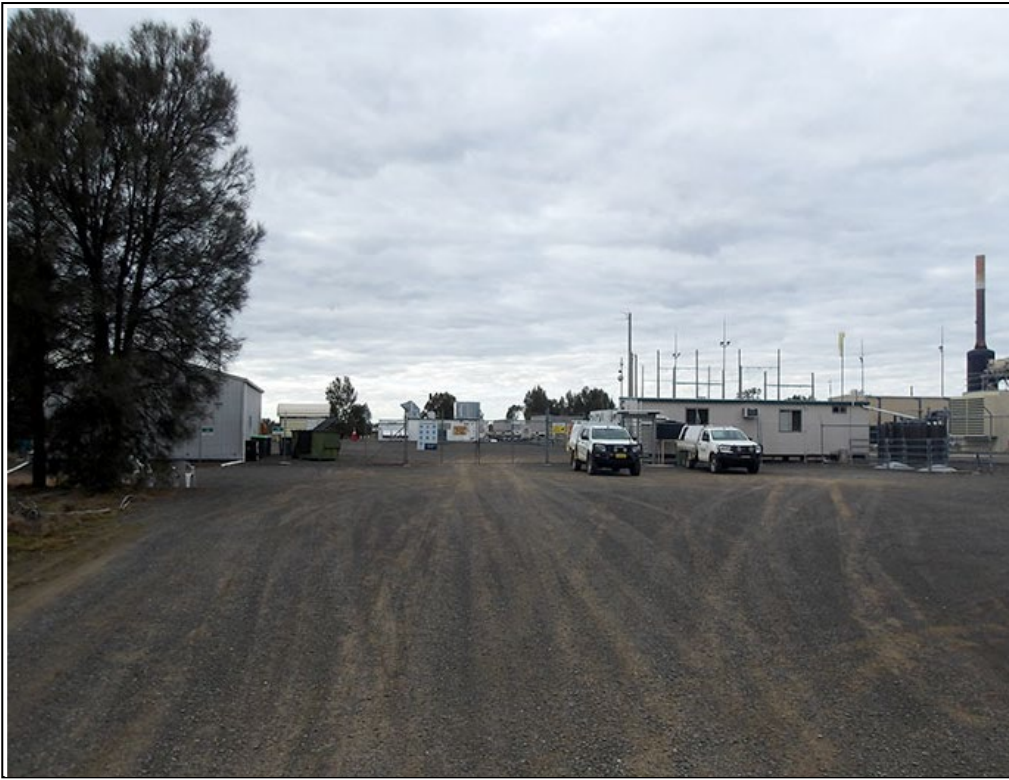
View east across Wilga Park Power Station entry way.
